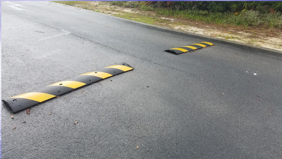
Speed Bumps on Radiant Circle
